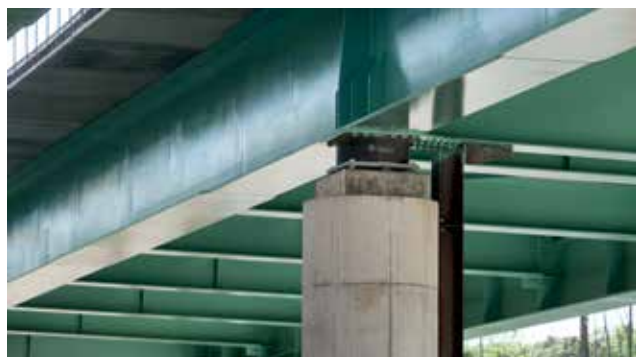
Pedemontana Motorway, Lura Viaduct (Italy)
